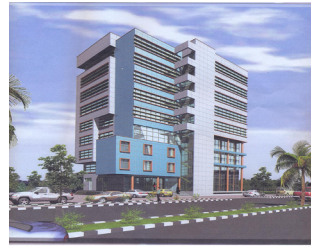
The new building of EFMHACA
